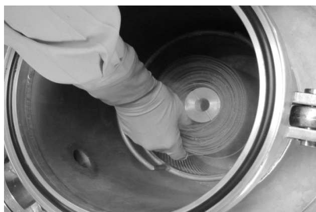
Fig. 11 Installation of irradiated nonwoven fabric to reaction vessel
