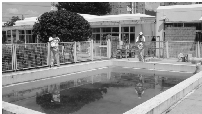
Fig.25 The swimming pool of kindergarten attached to Fukushima University
