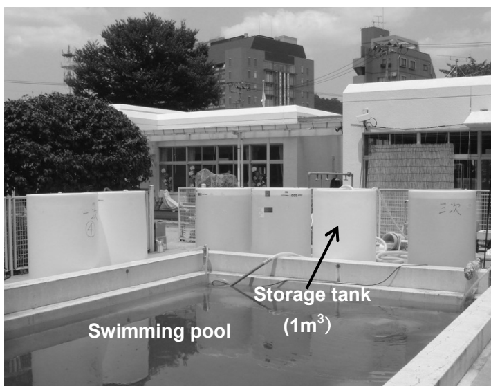
Fig.28 Storage tank installation scenery
